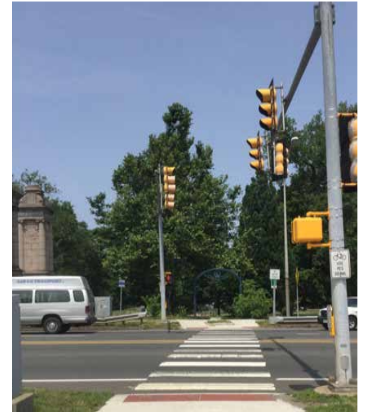
At the intersection of West Street and Riverside Road, a pedestrian countdown signal has been installed but no wayfinding signs are posted.
