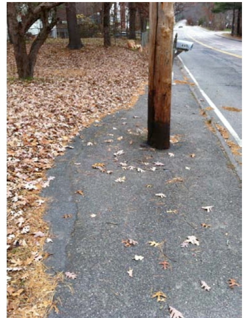
Expand the sidewalk with asphalt around utility poles.
