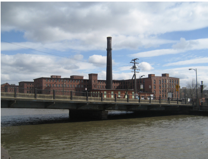
View of First-Level Canal and brick industrial buildings
