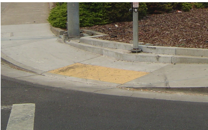
Curb ramp with detectable warning strip - sacdot.com
