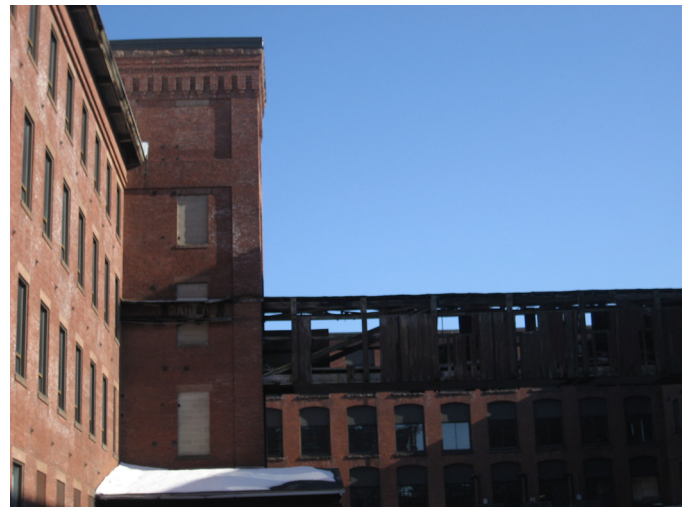
Industrial buildings ready for redevelopment
