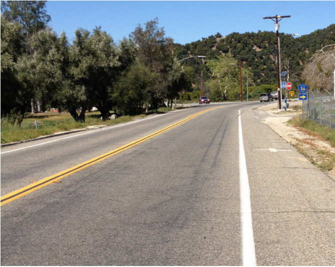
Fog lines delineate the vehicular driving zone on wide roadways.
