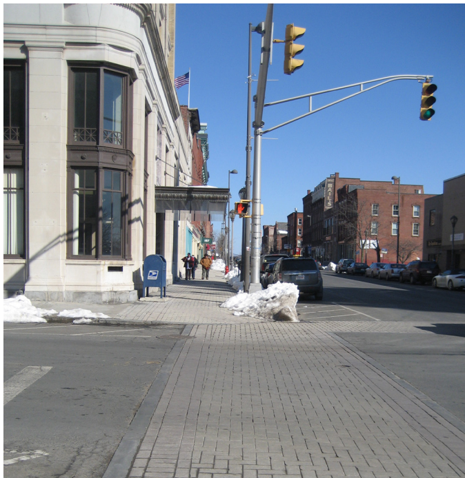
Concrete paver crosswalks at the Dwight Street and High Street intersection
