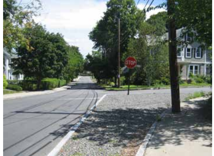
(A) Gravel-filled curb extension
