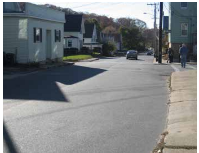
Narrow, uneven sidewalks along this stretch of Baker Street present challenges for many walkers.
