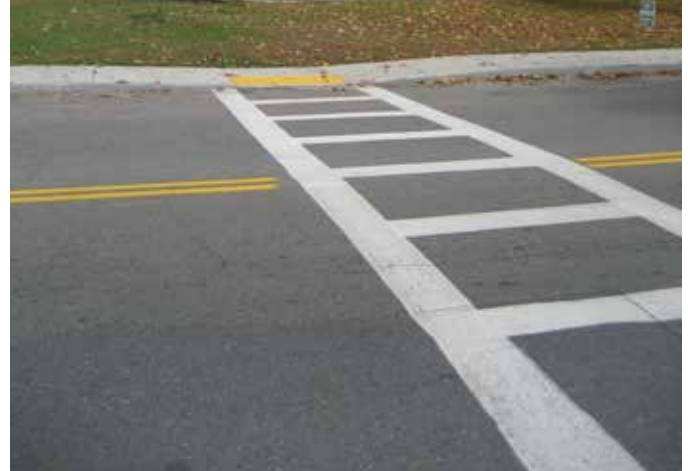
Crosswalks, curb ramps and detectable warning strips were recently upgraded along Parker Street.
