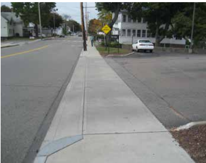
The GFA Federal —Credit Union driveway is excessively wide with four lanes of traffic proceeding across the sidewalk.
