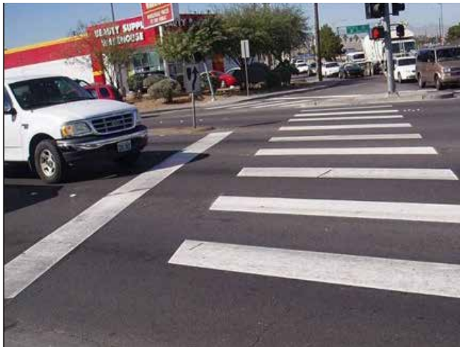
Crosswalk and stop line Source: http://safety.fhwa.dot.gov/ped_bike/tools_solve/ped_scdproj/sys_impact_rpt/images/fig16.jpg
