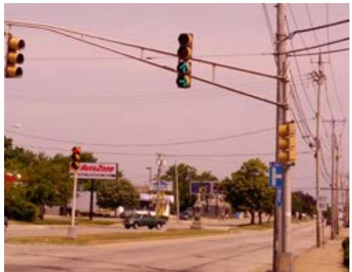
Signal that does not provide any walk time
