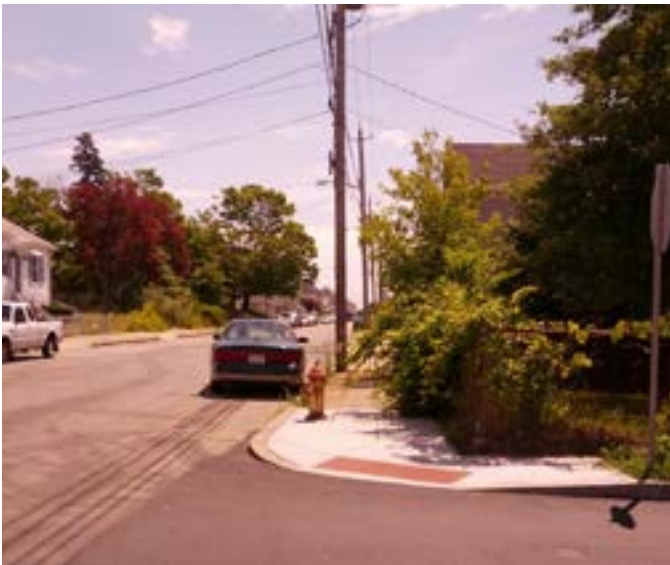
Curb cut blocked by overgrown shrubs
