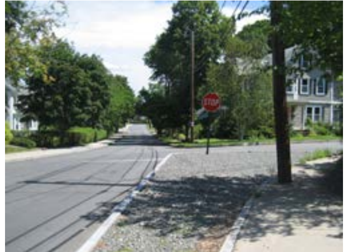
(A) Gravel-filled curb extension
