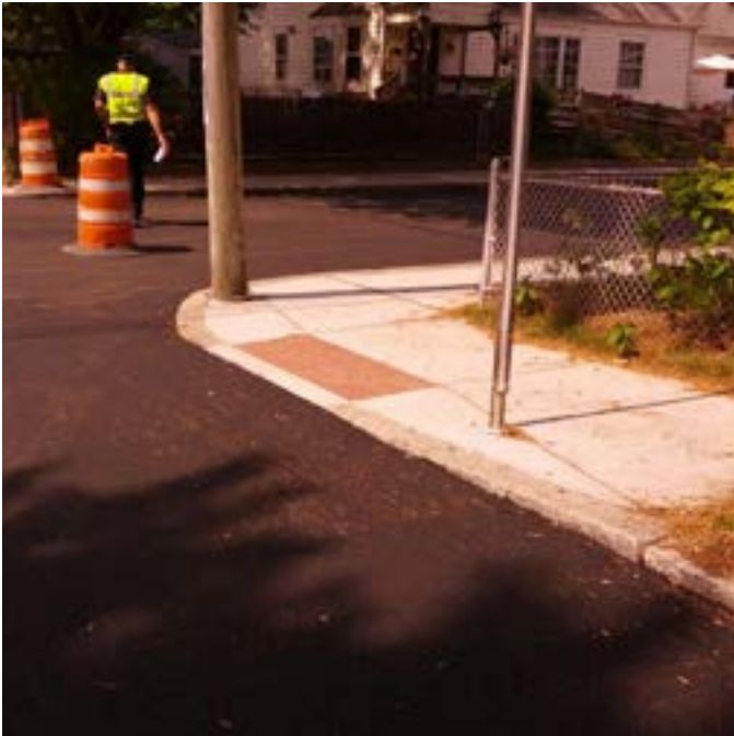
New curb ramp being installed in neighborhood
