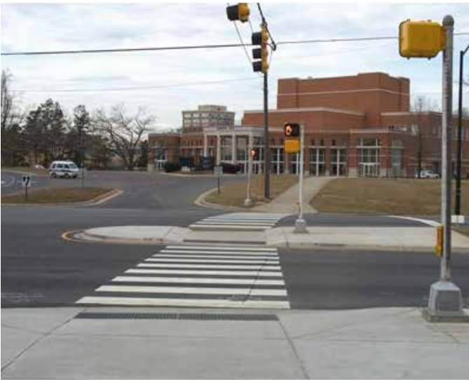
Pedestrian refuge island at a signalized crossing Source: http://safety.fhwa.dot.gov/intersection/resources/fhwasao6o16/images/fig95.jpg
