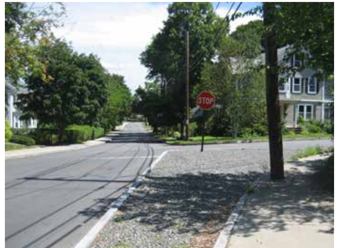
(A) Gravel-filled curb extension
