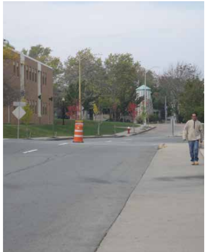
In-street pedestrian traffic barrel draws attention to crosswalk on N 6th Street connecting a parking lot used by Post Office employees to the Post Office
