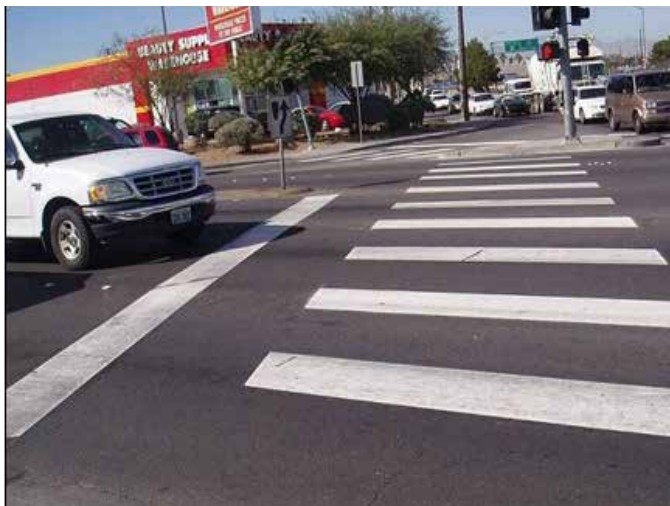
Crosswalk and stop line Source: http://safety.fhwa.dot.gov/ped_bike/tools_solve/ped_scdproj/sys_impact_rpt/images/fig16.jpg
