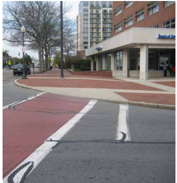
Wide curb radius at northeast corner of Pleasant Street/Elm Street intersection
