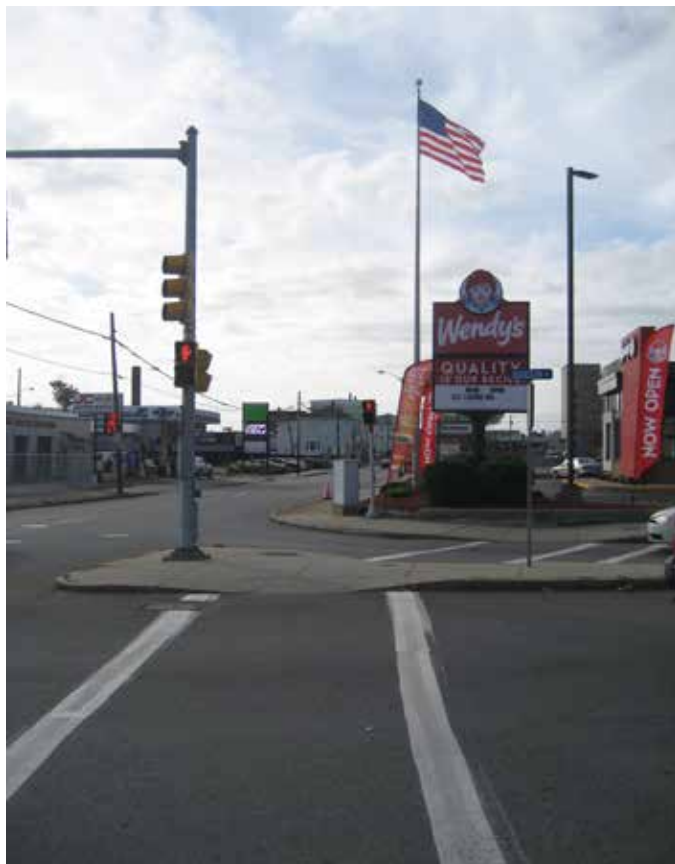
Pedestrian crossing on Robeson Street where WALK signal lights are out.
