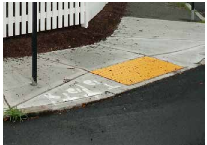
Curb ramp and detectable warning strip in Woburn, MA
