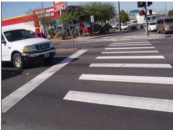
Crosswalk and stop line Source: http://safety.fhwa.dot.gov/ped_bike/tools_solve/ped_scdproj/sys_impact_rpt/images/fig16.jpg
