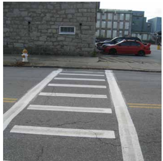
Missing curb ramp and detectable warning strips on Robeson Street
