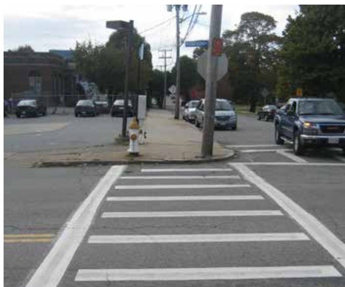
Non-ADA compliant curb ramps on Robeson Street and Pine Street
