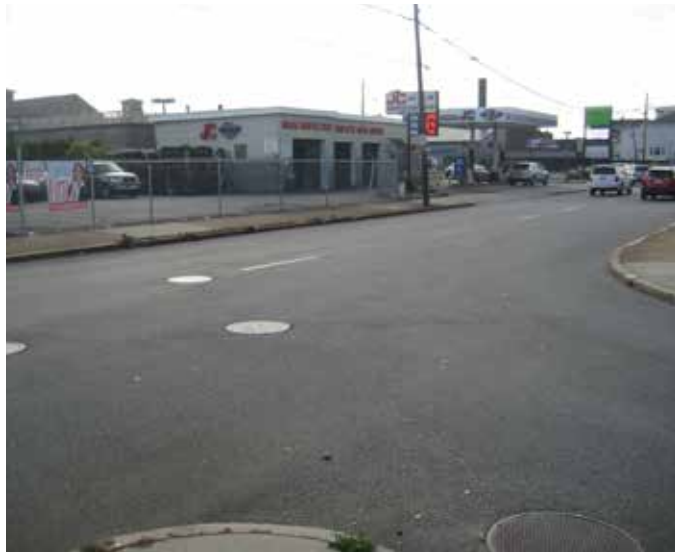
Absence of a pedestrian crossing along 12th Street
