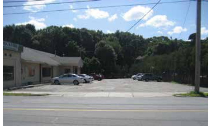
The curb cut leading to the Dockside Restaurant is excessively wide facilitating fast turns into the parking lot and extending the time pedestrians are in a potentially dangerous position.
