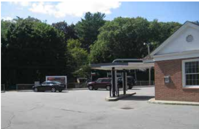
Pedestrian and vehicular zones should be clearly marked to avoid conflicts when accessing the T stop.
