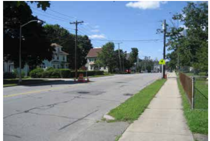
Pedestrian crossing signs in advance of the Greenwood School would increase driver awareness of pedestrians in the area.
