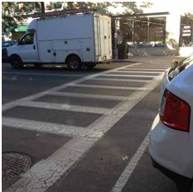
Curb bump-outs would increase pedestrian visibility at this mid-block crossing on Washington Street
