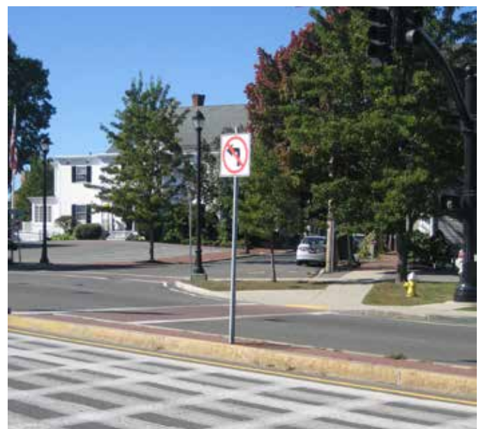
Upon observation, pavement markings and traffic median and sign do not manage traffic effectively at this intersection.
