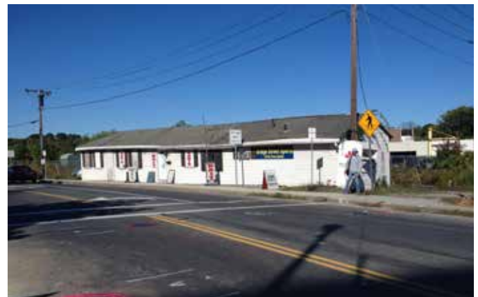
Crosswalk pavement markings on Bridge Street are minimal
