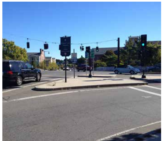
This right turn slip lane from Bridge Street onto Washington Street is confusing to pedestrians and drivers - it is unclear who has the right of way
