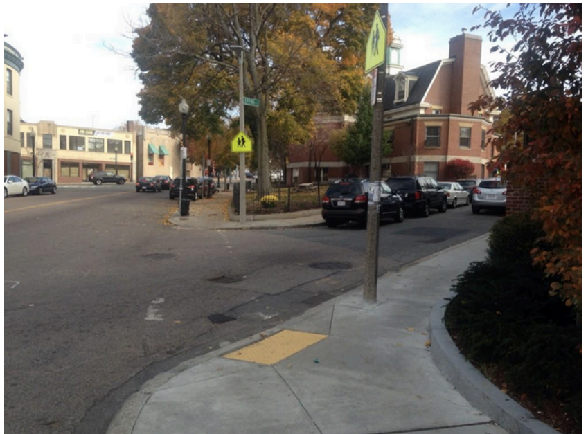
Wide turning radius from Norfolk Street onto Epping Street with faded crosswalk. Front door to Codman Academy is on the right.
