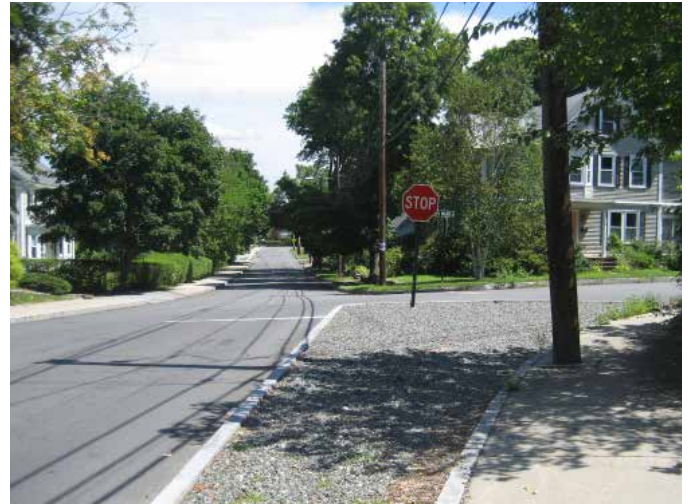
(A) Gravel-filled curb extension
