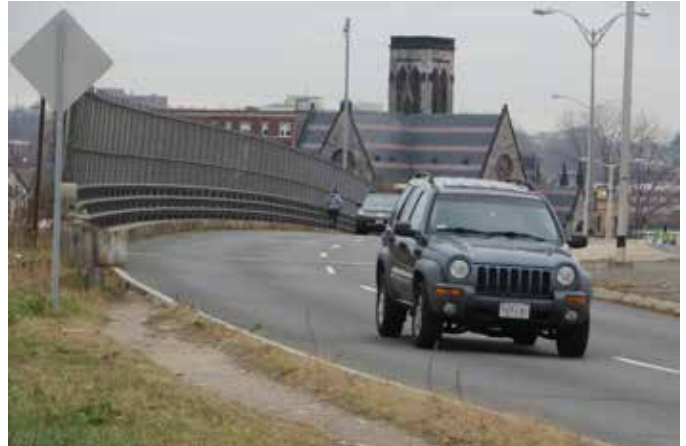
A lack of pedestrian facilities at the convergence of the Birnie Avenue ramp with Route 20/Plainfield Street leads to risky and unsafe pedestrian and bicyclist behavior.
