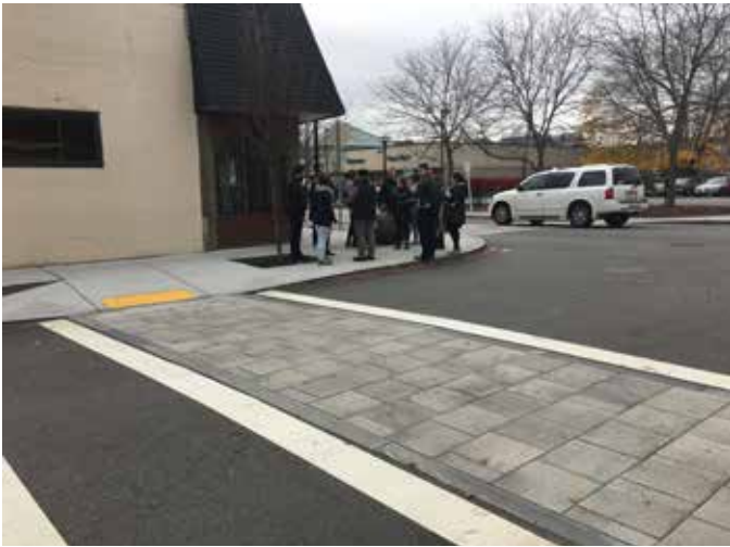
New crosswalk designs just south of the study area include pavers, transverse lines, and detectable warning panels
