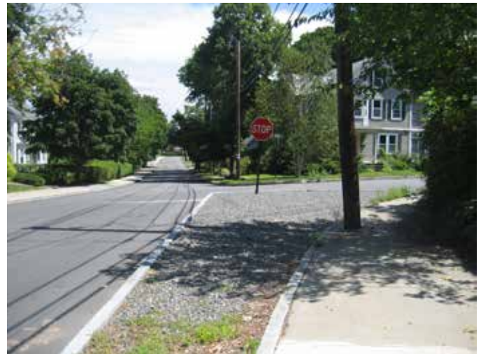
(A) Gravel-filled curb extension
