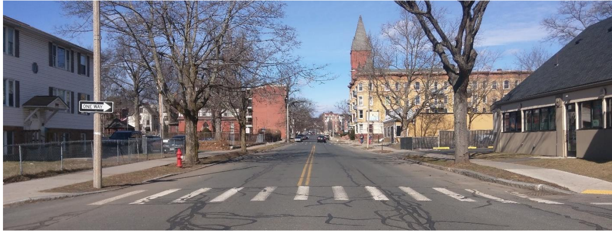
Image 6: Appleton Street Corridor facing eastbound.
