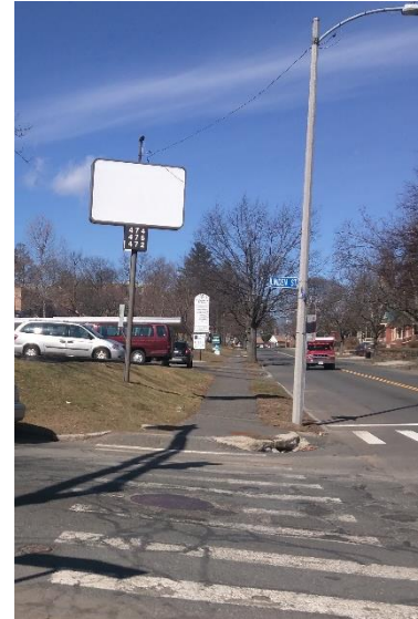
Image 9: Asphalt sidewalks on the south side of Appleton Street north of Linden Street.
