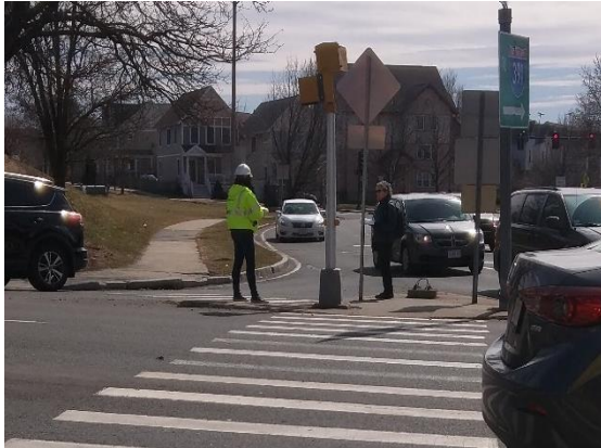
Image 4: Splitter island on Resnic Boulevard northbound approach with pedestrian signal heads rotated and missing light pole.
