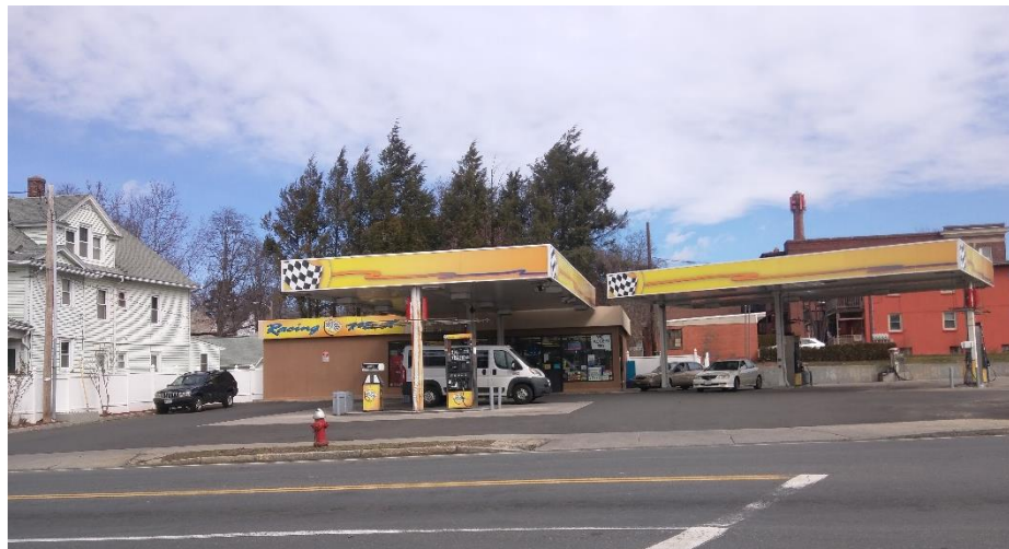
Image 5: Curb cuts on W Franklin Street at gas station.
