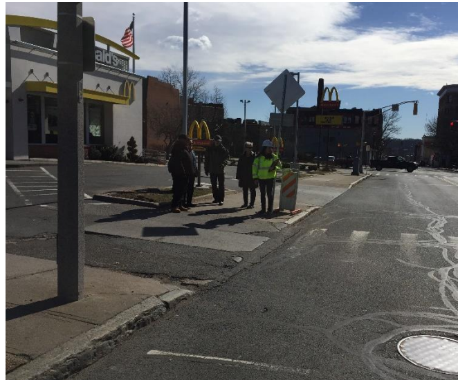
Image 14: Faded crosswalk located within McDonald's driveway on Appleton Street east of Chestnut Street.
