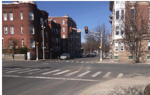
Image 10: Missing crosswalk on north east leg of intersection of Appleton Street at Beech Street.
